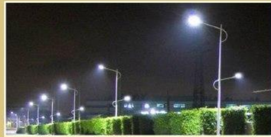
Electrical Lines With Designer Street Lighting
